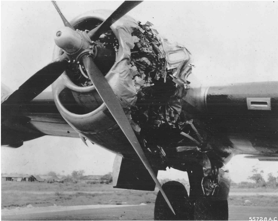
Fig. 15 The crew of this Boeing B-29 was able to feather the propeller and get safely home.
